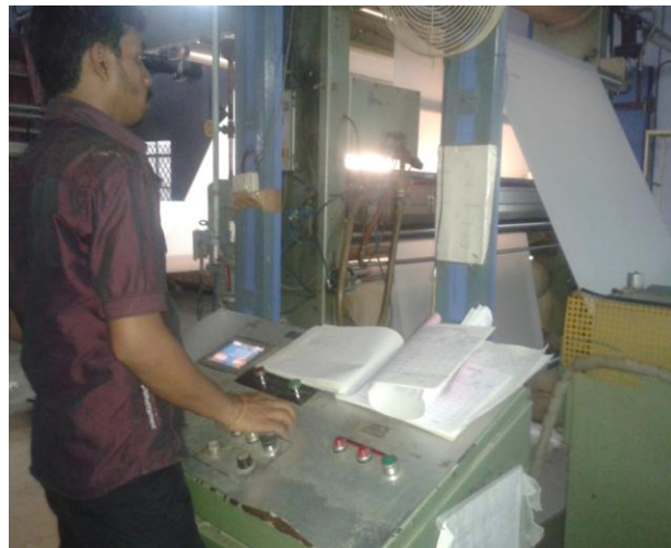
operating of main panel board
